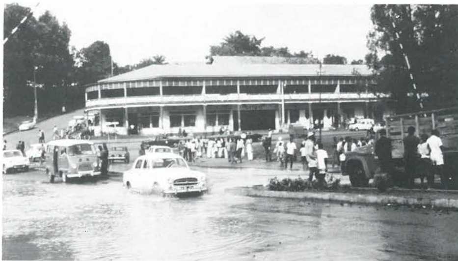
Yaoundé : flooding in the railroad station area
