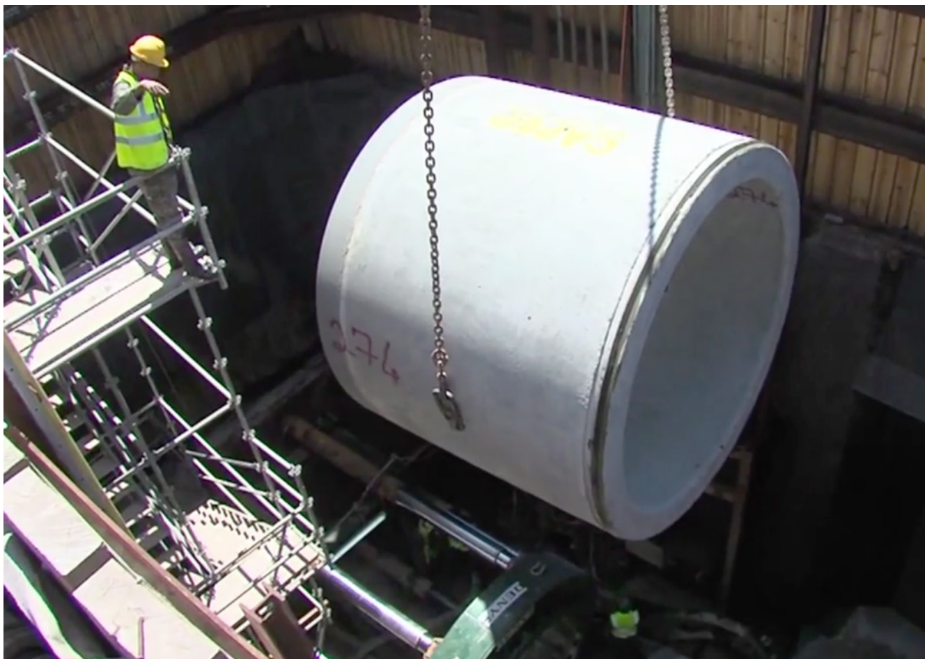
Laying a main sewer in a wastewater treatment plant in Greater Casablanca
